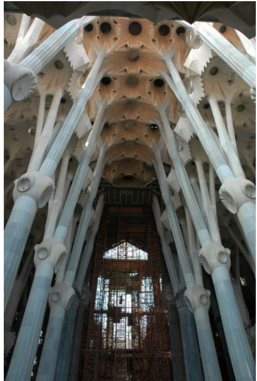
View of interior columns
